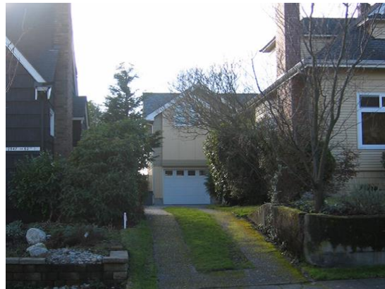
Image Source: City of Seattle, Department of Planning and Development: Backyard Cottages Annual Report (2014).
