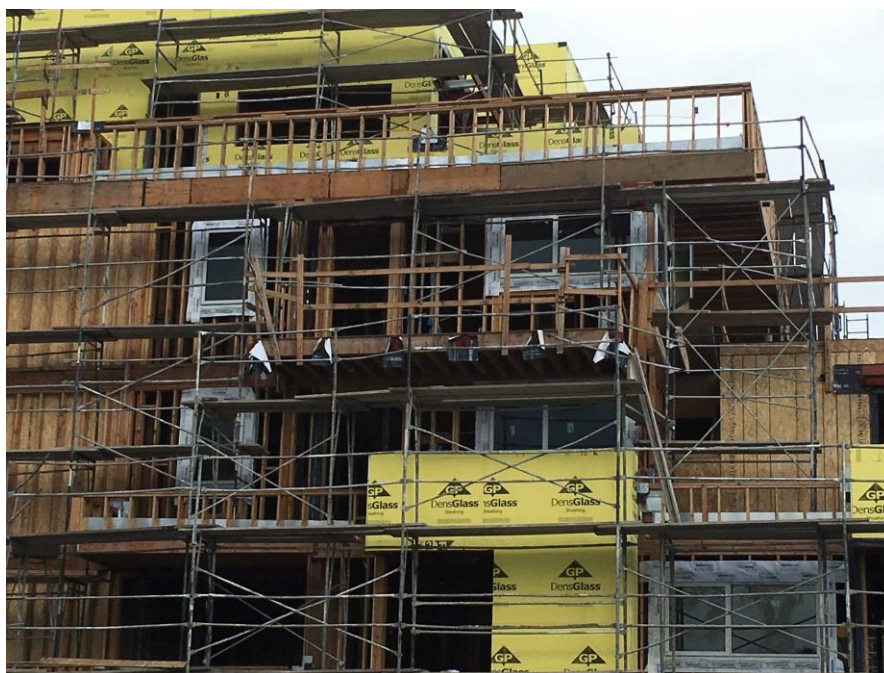
Picture of Apartment Under Construction Image source: Personal Image
